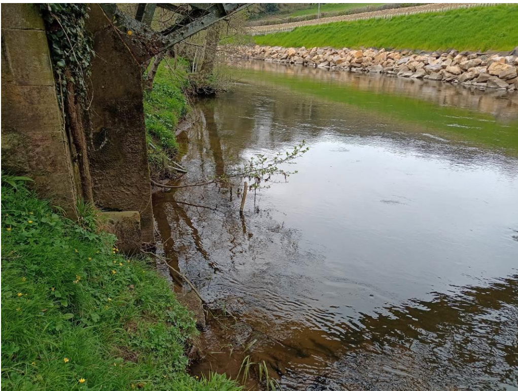
Photo 7 Hard-engineered left (far) bank and sewer storm overflow pipe (foreground).
