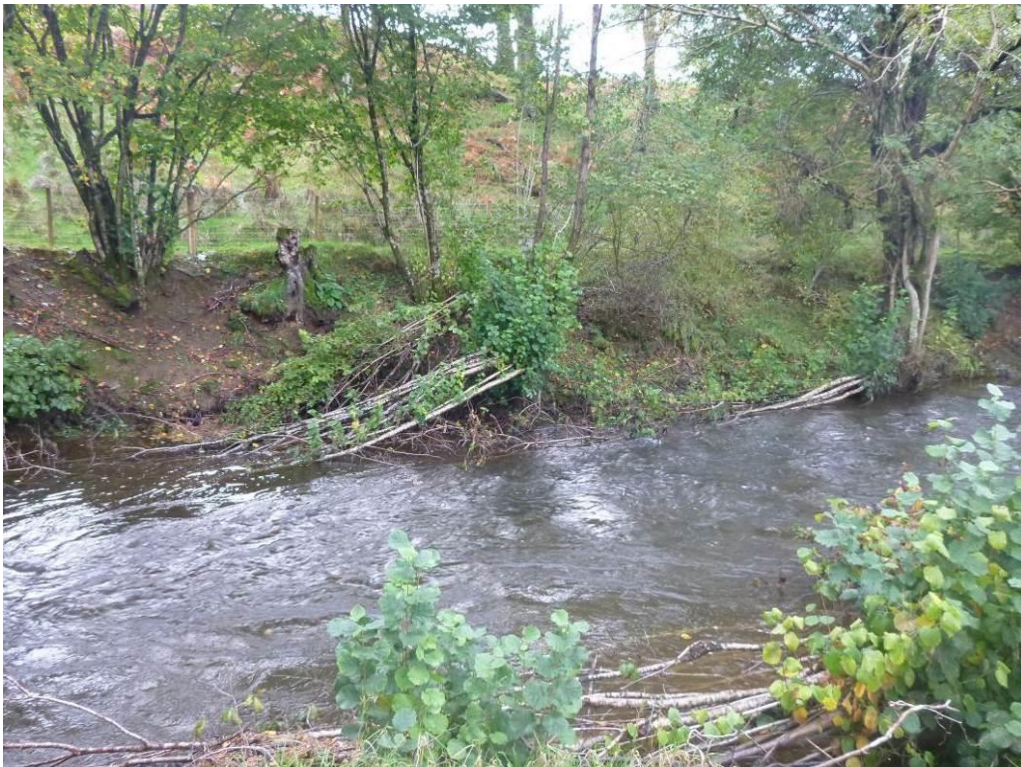
Photo 9 Laying small trees/coppice re-growth to provide low cover in/over the river.
